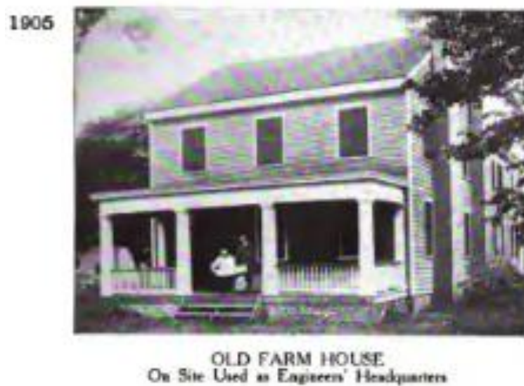
Figure 4. Undated Photograph Showing Domestic Structure in Likely Vicinity of Current N26 and 44NR0036. Demolished prior to Jamestown Exposition in 1907 (Source: The Official Bluebook of the Jamestown Ter-Centennial Exposition (1909:77))
